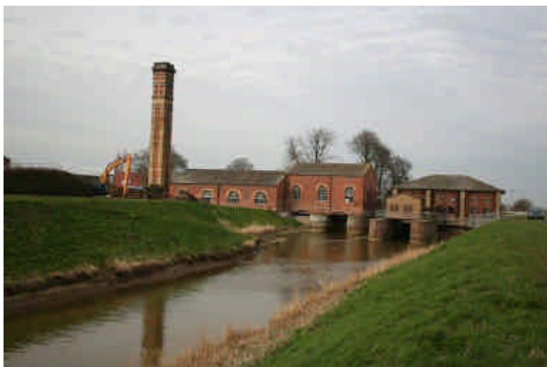
Lade Bank Pumping Station ©Richard Croft
